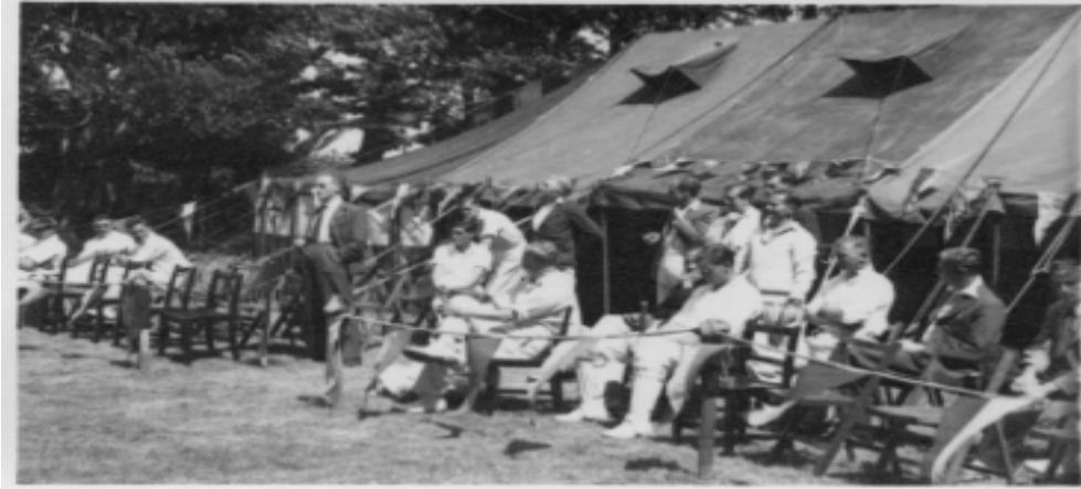
Opening of the ground – S.R.D.E Christchurch – Saturday 9 th July 1949
